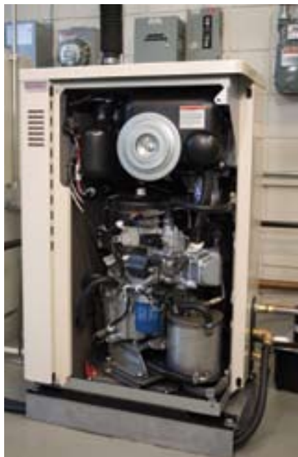
Figure 8. Combined heat-and-power (CHP) generation can now take place in the home. This micro-CHP system, manufactured by Honda, produces 3.26 kilowatts of heat and 1.2 kilowatts of electric power. The electricity is generated as a byproduct of heating, which also leads to reductions in the generation of carbon dioxide from heating. In certain states, homeowners are allowed to sell any unused power generated back to the electrical grid in their community. A similar micro-CHP system has been on the market in Japan since 2003, with more than 45,000 units sold there to date. Image courtesy of American Honda Motor Corporation.
